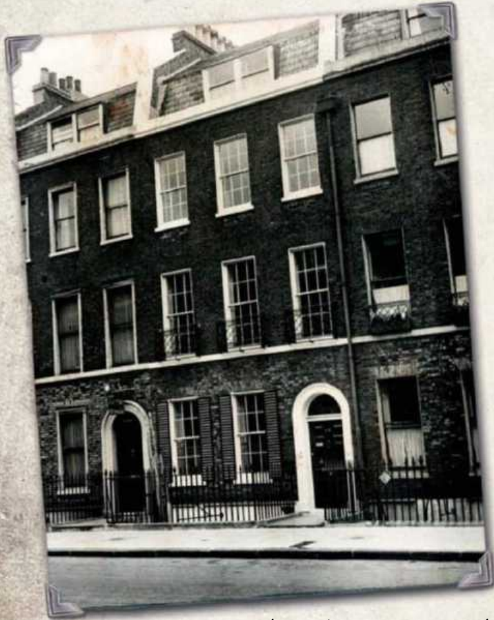
The Baker Street House had been empty for some time.
